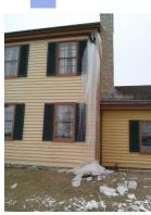
For the second winter in a row, the Colonel Davenport House has experienced large ice dams when thick ridges of solid ice build up along the eaves. Because of faulty routing of the furnace/air conditioning condensate removal piping, the water from the system cannot be dumped directly outside. We have a plan that will allow the routing of the condensate piping directly into the house drain without going outside.
